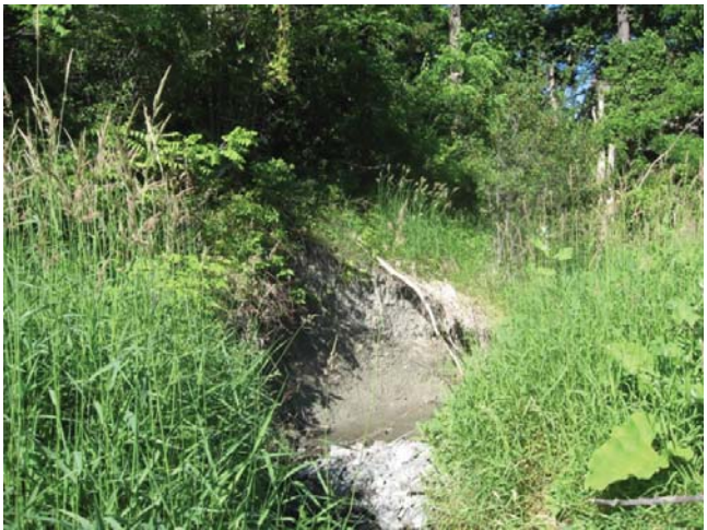
Photograph 12. ↑ Scour on left bank, downstream of crossing
